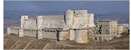
12th-century Knights Hospitaller castle of Krak des Chevaliers in Syria, one of the first castles to use concentric fortification, i.e. concentric rings of defence that could all operate at the same time. It has two curtain walls and sits on a promontory.
